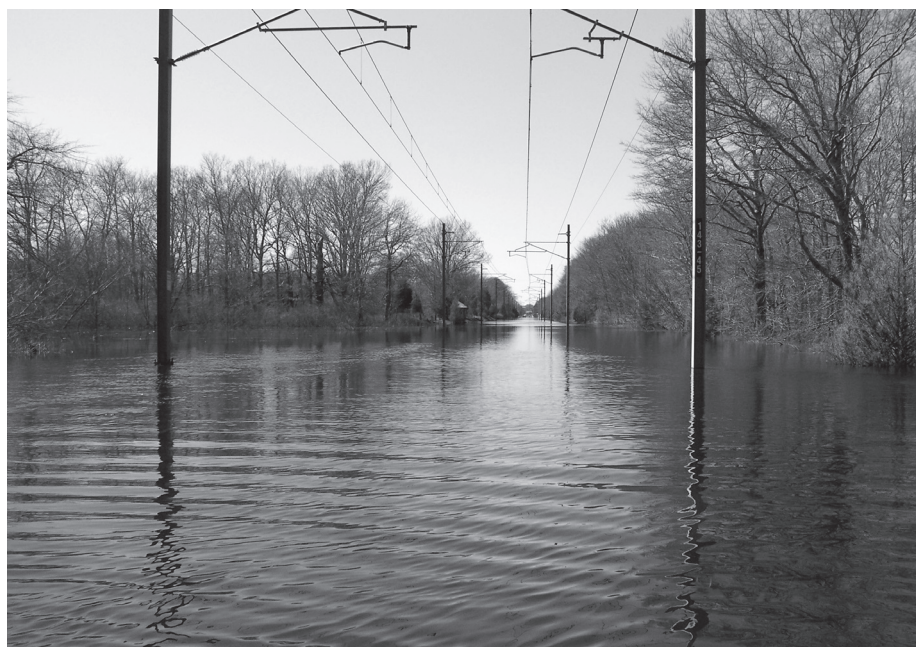
Floodwaters, 16 inches deep in spots, cover Amtrak's Northeast Corridor line passing through Rhode Island's Great Swamp, four miles south of the Kingston station, on April 1. Photo by Richard Neff, Jr. Amtrak
