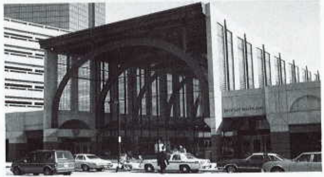
For many travelers, beautiful new Back Bay Station (Oct.-Nov. News, p. 3) will be the most convenient Amtrak station in Boston. The building, designed by Kallmann, McKinnell & Wood for the Massachusetts Bay Transportation Authority (MBTA), is located at 145 Dartmouth Street. In addition to Amtrak intercity trains, the station is served by MBTA commuter and transit (Orange Line) trains. The station's waiting room is dedicated to A. Philip Randolph (1889-1979), civil rights leader and founder of the Brotherhood of Sleeping Car Porters union.
